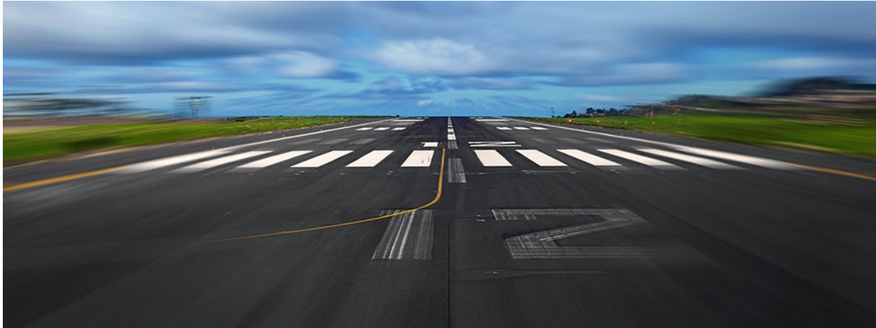
Figure 4 - Airport runway [Image credit: aertecsolutions.com, https://bit.ly/2LOtFJE ]
